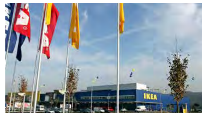
General planning of the building technology, heating, air conditioning, sanitary facilities, new IKEA building, Spreitenbach
