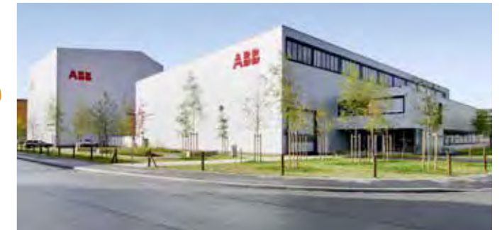
ABB: new production plant and laboratory building for high voltage switchgear; Helbling Beratung + Bauplanung planned the entire building technology
