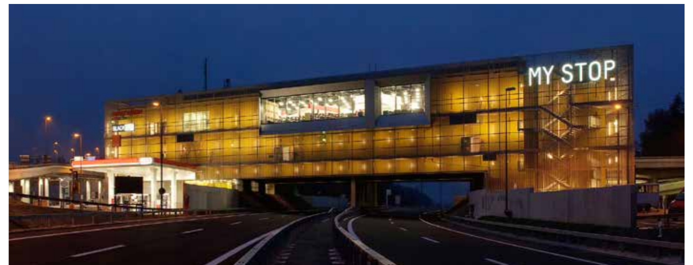
Planning of building technology for MY STOP, highway service station Affoltern am Albis
