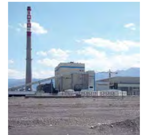
Engineering of Air Cooled Condenser (ACC) for thermal power plant Shengxiang 2x330 MW in China
