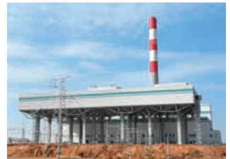
Air-cooled condensers of Qingtongxia thermal power plant (2 x 330 MW), China
