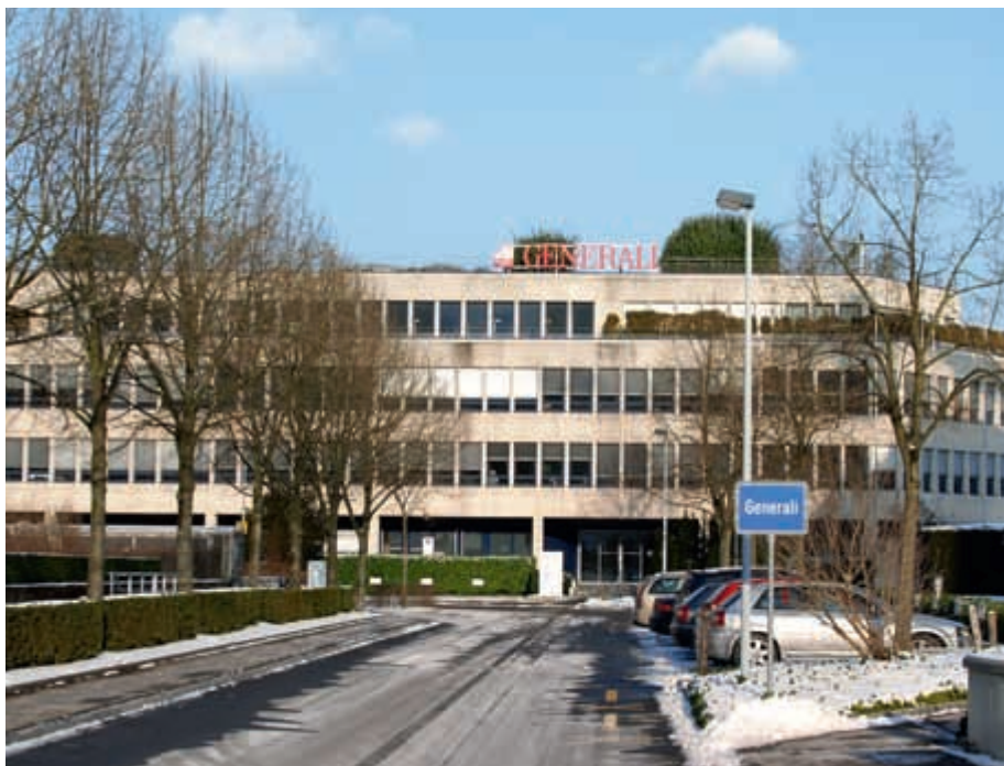
Head office of Generali Switzerland Insurance: general planning of the refurbishment of the data center
