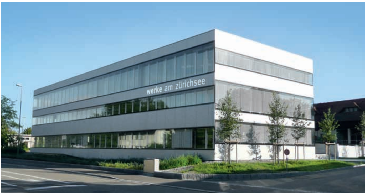
New works area/office building in Küsnacht for three communities: construction owner representation
